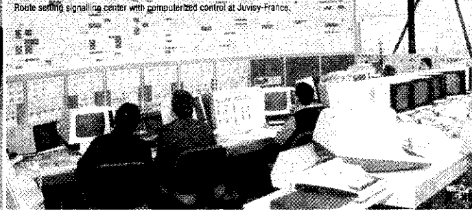
Route setting signalling center with computerized control at Juvisy-France.
